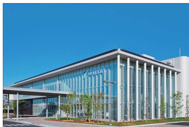
The Integrated Production Center at the Company's Kashima Plant aims to improve quality and productivity by integrating all of its people, organizations, and information
