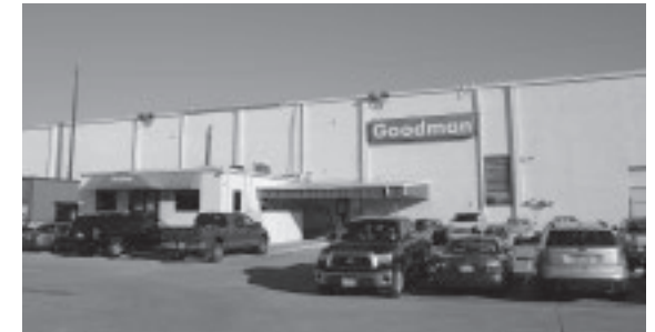
Goodman's Cooling Factory
