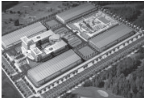
McQuay China, Wuhan Factory (top) Suzhou Factory (left)
