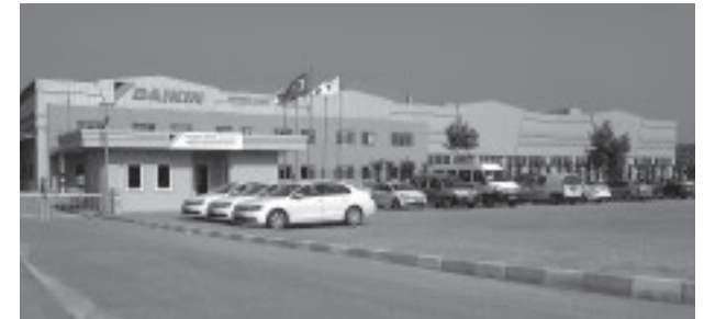
Hendek Factory of Daikin Turkey A.S.
