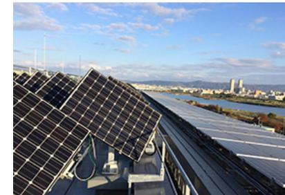
Solar power generation system has panels that move to track the sun's position (at TIC)
