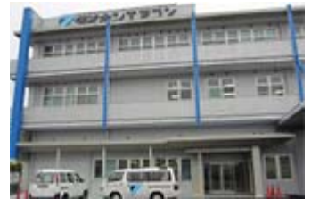
New plant of Daikin Sunrise Settsu
