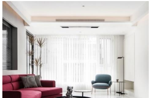
Installation example of downward airflow for indirect lighting
