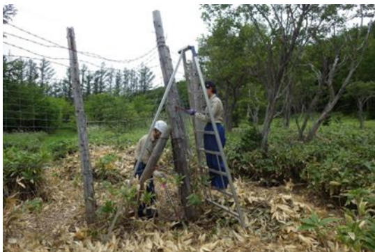
Photo 1-3: Repairing an aging deer fence (August 26, 2018)
