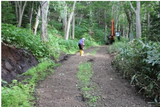
Photo 1-5: Smoothing out a service road (July 2, 2018)
