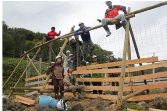
Photo 1-8: A completed deer fence (September 22, 2018)
