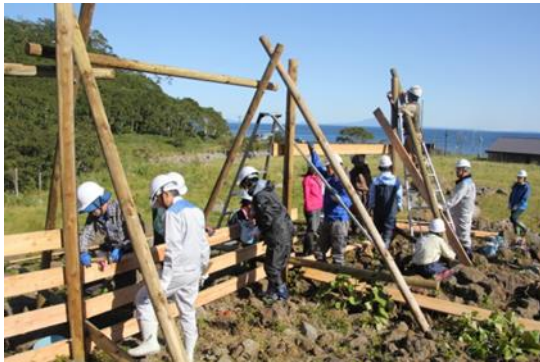
Photo 1-7: Erecting a deer fence (September 21, 2018)
