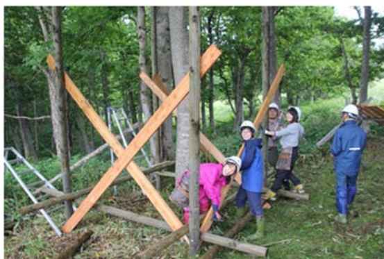
Photo 2-7. Tree deck installation at the work camp in July (July 6, 2019)
