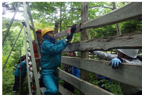
Photo 1-8. Repair of deer fence (September 20, 2019)
