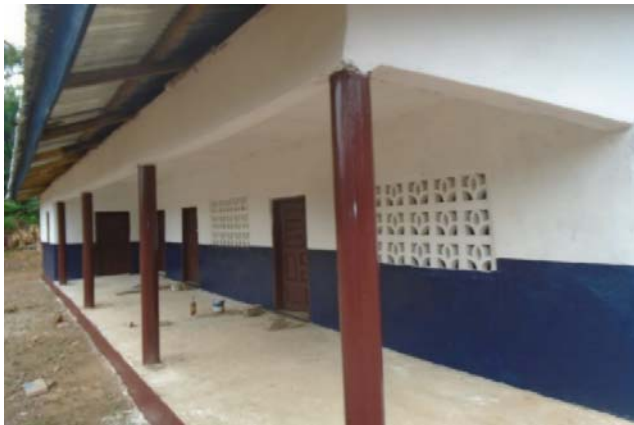
Elementary school renovation in Yolowee
