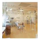
Collapsible negative pressure booth with aluminum frame
