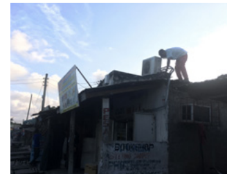
Installing an outdoor unit on a house
