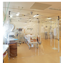
Collapsible negative pressure booth with aluminum frame
