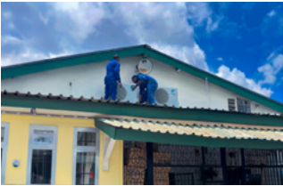
Installing an outdoor unit on a house
