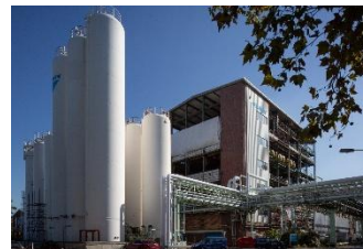
Refrigerant Regeneration Plant (Germany)
