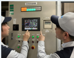
Checking for heat loss in real time
