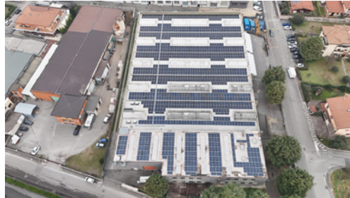
Daikin Compounding Italy S.p.A. introduced solar power generation system at its factory
