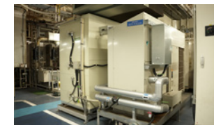
JIZAI HEAT installed at the Rinkai Factory
