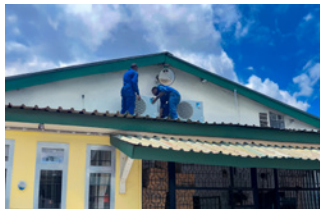
Installing an outdoor unit on a house
