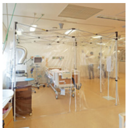
Collapsible negative pressure booth with aluminum frame
