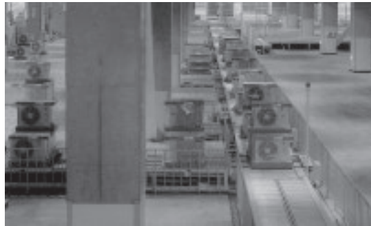
Automatic Materials Handling Equipment Inside Soka Center
