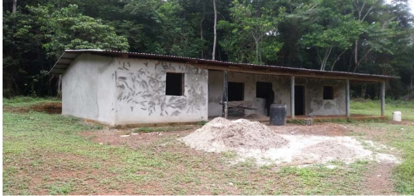
Yolowee school being renovated
