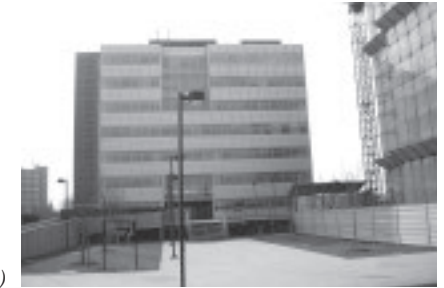
Daikin Airconditioning Italy (DACI)
