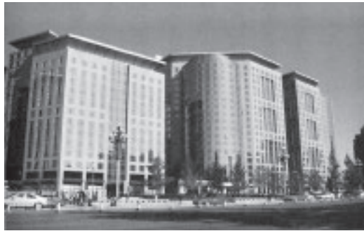
Beijing Headquarters of Daikin Investment (China) Co.
