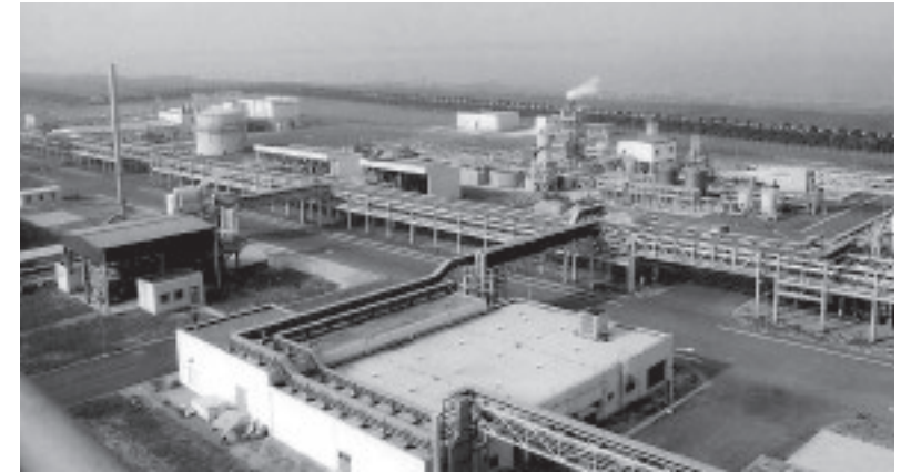
Jiangsu Plant of Daikin Fluorochemicals (China)
