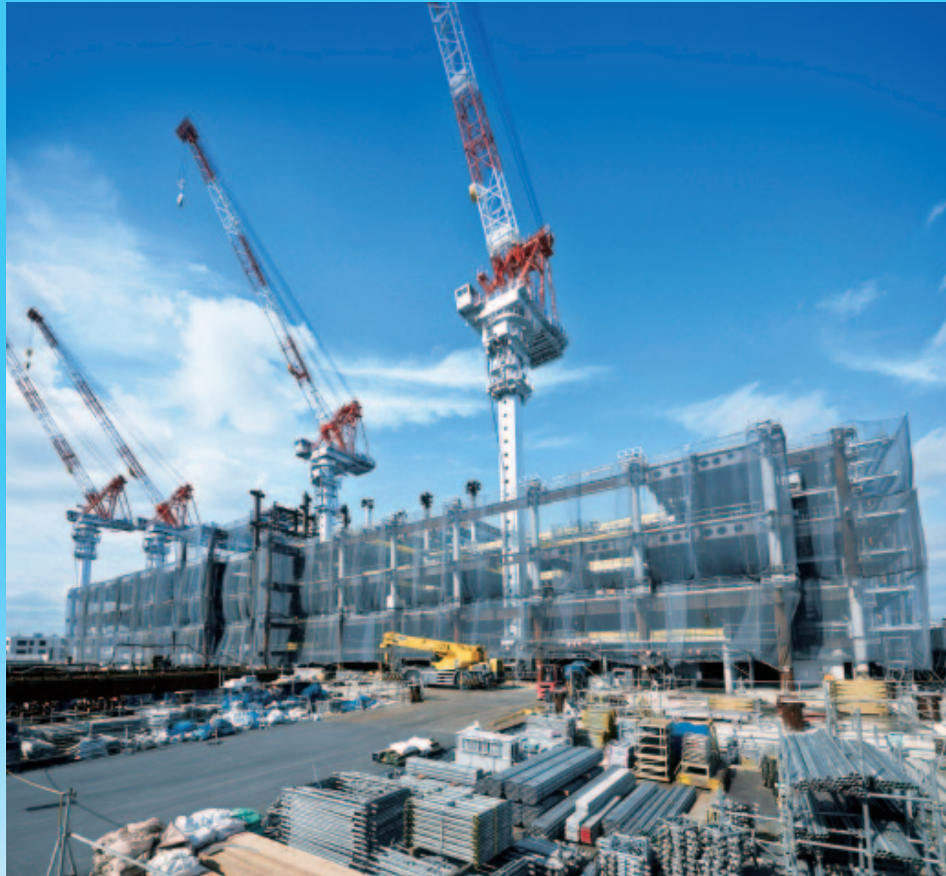
Technology and Innovation Center under construction
