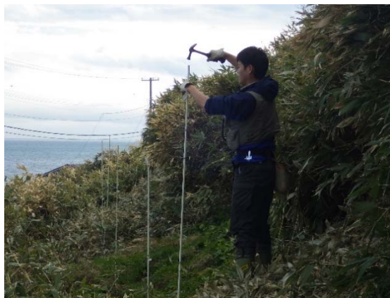
Photo 2-7. Installation of electric fences
