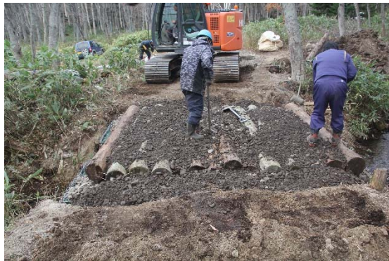
Photo 1-5. Ponthoro Bridge undergoing replacement work (November 6, 2020)
