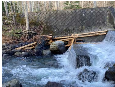
Photo 1-8 Damages incurred by the fishway on Banno River (November 11, 2021)
