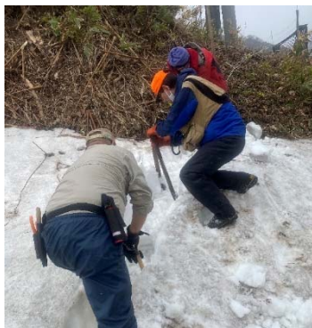
Photo 2-7. Installation of electric fences
