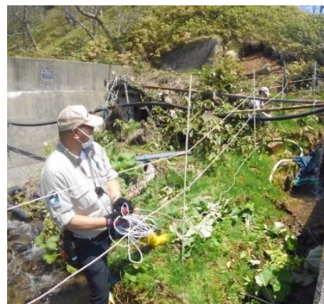
Photo 2-8. Installation of electric fences
