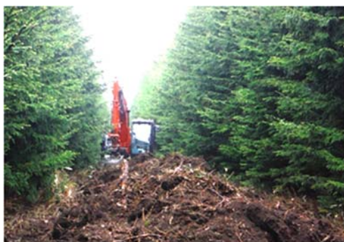
Photo 1-1. Removing broadleaf bamboo with heavy machinery (June 8, 2021)
