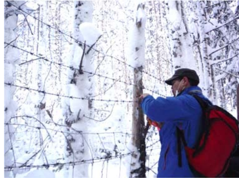
Photo 1-6 Repair work on deer fences (February 29, 2022)
