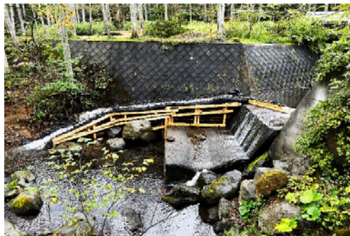
Photo 1-7 Progress of work on the fishway at Banno River (September 28, 2021)
