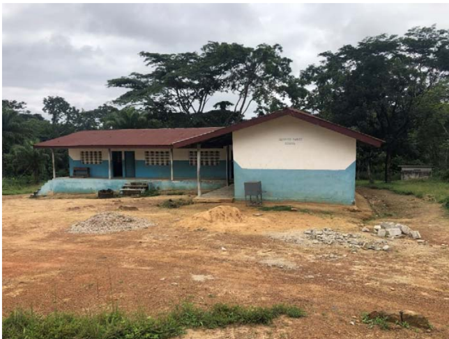
Public School renovated through assistance extended by the project © CI Liberia/Photo by George Ilebo
