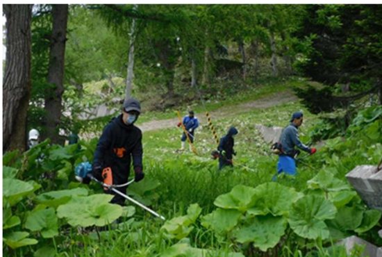
Photo 3-5. Local residents and company employee volunteers clearing bushes to create an open space
