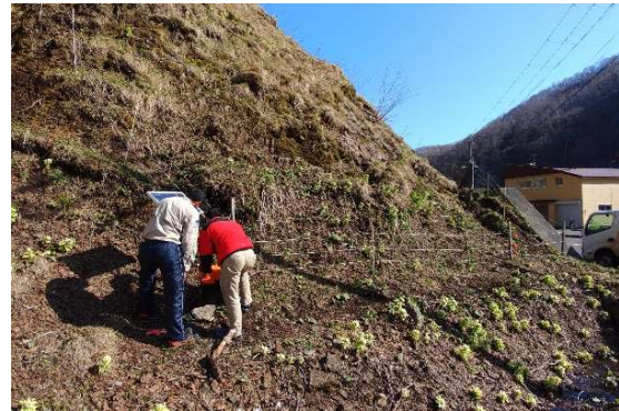
Photo 3-2. Installation of electric fences
