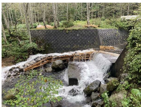
Photo 1-5. Simple fishway on the Banno River after repair (October 11, 2022).
