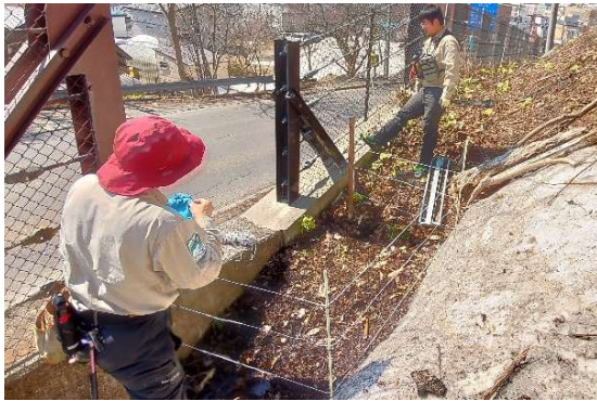
Photo 3-1. Installation of electric fences
