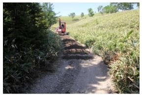
Photo 1-6: Repairing a service road (June 19, 2018)
