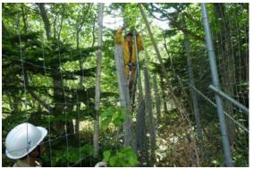
Photo 1-5: Pile driving work (June 22, 2018) on the steel deer fence posts (repair on fence erected in 2003)
