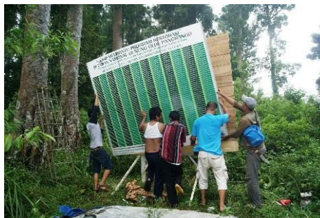
Repairing one of the signboards
