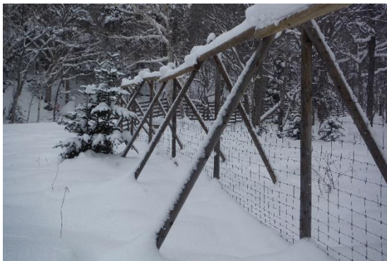
January: This deer fence along the Iwaobetsu River was reinforced in autumn 2016
