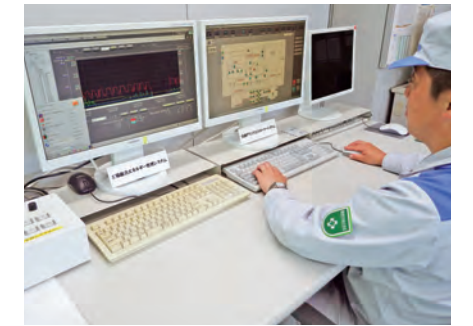
D-BIPS* and other methods are used to control all energy used at the plant, make visual representations of energy usage, and develop energy-saving activities for all divisions
